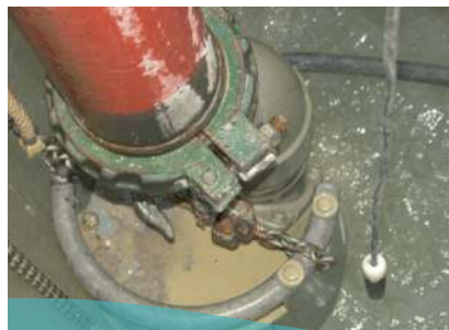
Building site pumps
